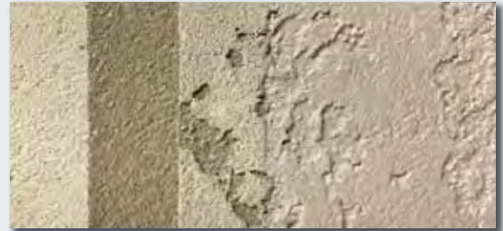
Primer Slurry Knockdown Color and Seal Texture
